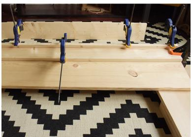
3. Next, use RapidFuse to adhere a 1" x 4" x 4' board to the 1 x 12, butted up against the 1 x 2 board, as shown and clamp together until dry.
