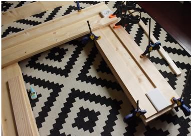
8. Glue the plinth block next to the 1 x 4 x 3' board. Then glue another 1 x 4 board, butted up next to the finnial, as shown. Do this on both legs.
