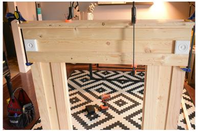
10. Use RapidFuse to adhere the 1" x 6" x 4' board to the top, making sure the back edge is aligned with the back edge of the fireplace. Clamp in place until dry.
