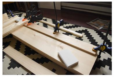
7. Glue a 1  $\times$  4  $\times$  3' board to the edge of one side of the fireplace leg. Clamp together until the glue is dry.
